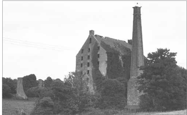
Ballydugan mill, derelict before its restoration by Noel Killen. The flour mill was built in 1792 by a company owned by John Aughinleck of Strangford. DJ41/877/01/01
